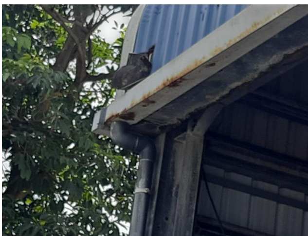
Rusted Gutter
