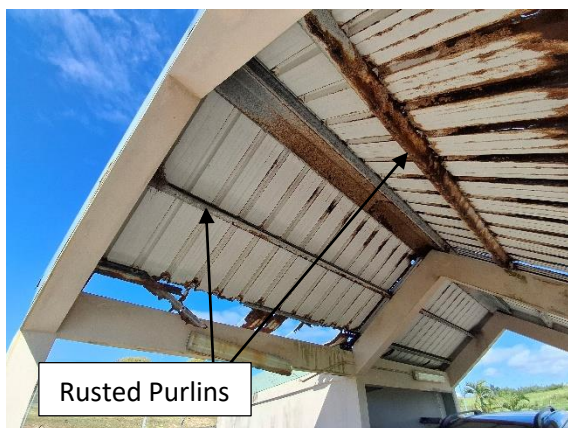
AIRCRAFT DISCHARGE SHED
