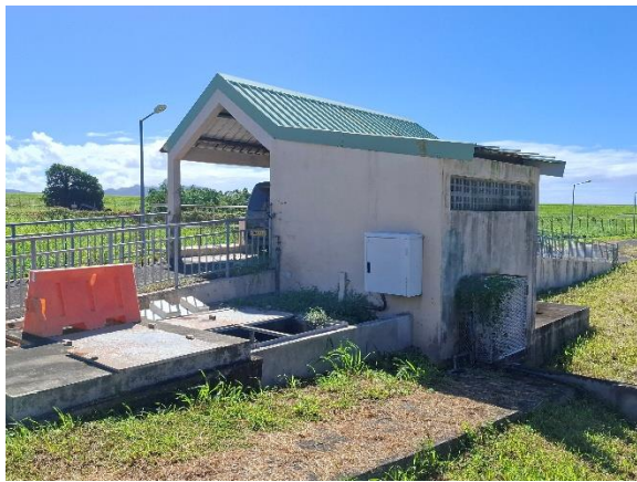
RHS ELEVATION ( Approx 6.0m from GL)
